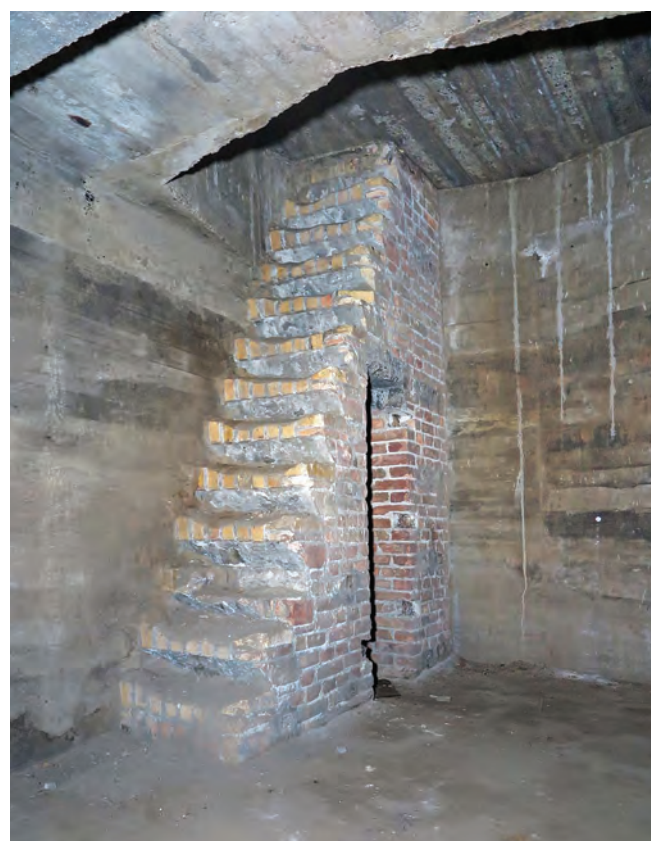
The wartime steps into the Tiergarten tunnel, heavily worn by factory workers and those seeking shelter. Photo Clive Penfold
